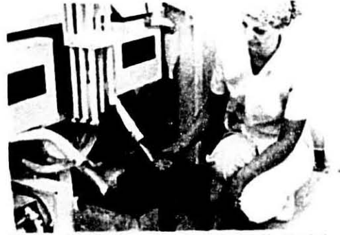
Experimental mills are used by International Multifoods to grind wheat samples into flour for pre-evaluation. The flour is made prior to large scale production.
